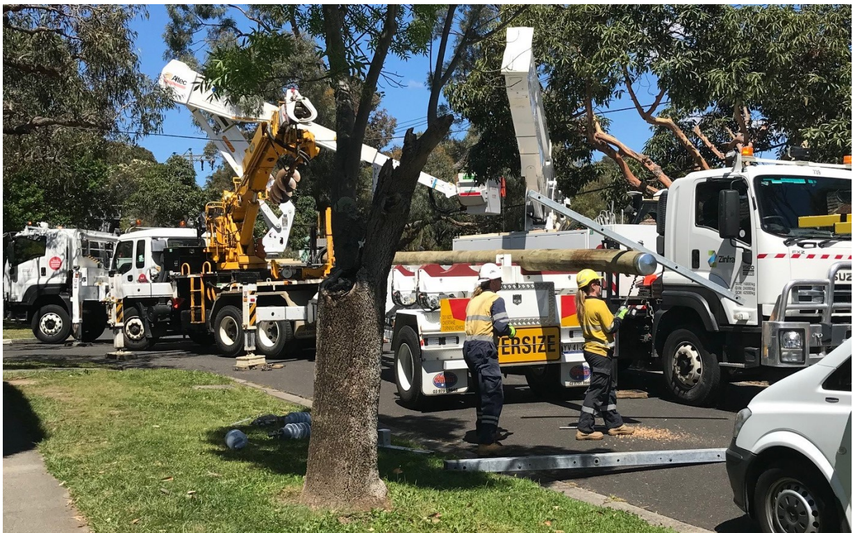
Responding to storm damage in Blackburn, 31 October 2021 (Source: IGEM)
